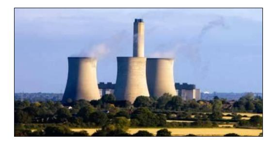
Didcot A Power Station is a dual-fuel (coal and gas fired) power station located in the civil parish of Sutton Courtenay, next to the town of Didcot in Oxfordshire (formerly in Berkshire). Construction commenced in 1964 in the face of local opposition from the village of Sutton Courtenay and the station commenced generating in September 1970. Didcot A has four generating units, each rated at 500MWe, giving the station a total generating capacity of 2000MWe.
